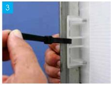
Fit the back tabs over the solid fin of the star picket.
