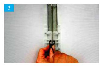
Refit both signAclips to the star picket and position both clips over a single predrilled hole on the star picket. Insert a single cable tie through both clips and a predrilled hole and tighten the cable tie to secure both signs to the star picket.
