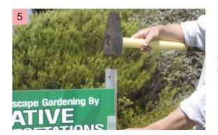
Holding the signAclip onto the picket, hammer the 2<sup>nd</sup> star picket to the same depth as the 1<sup>st</sup> one, locate a predrilled hole on the star picket and secure with a cable tie
