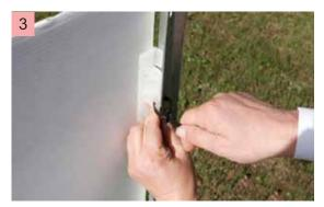
Refit the signAclip to the 1<sup>st</sup> star picket and position the clip over a single predrilled hole. Insert a single cable tie through the clip and the predrilled hole. Tighten the cable ties to secure the sign to the 1<sup>st</sup> star picket.
