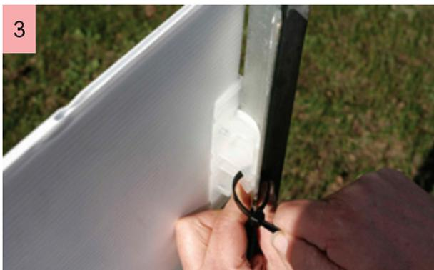
Refit the signAclip and position over a predrilled hole. Insert a cable through both the clip and the predrilled hole and tighten the cable tie to secure the sign to the star picket.
